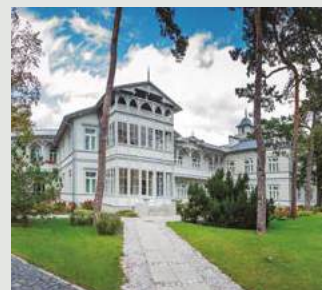
Gurewicz Spa Resort. Hotel- Restaurant - Spa. Otwock, Poland. PACi, VRF and Control.
